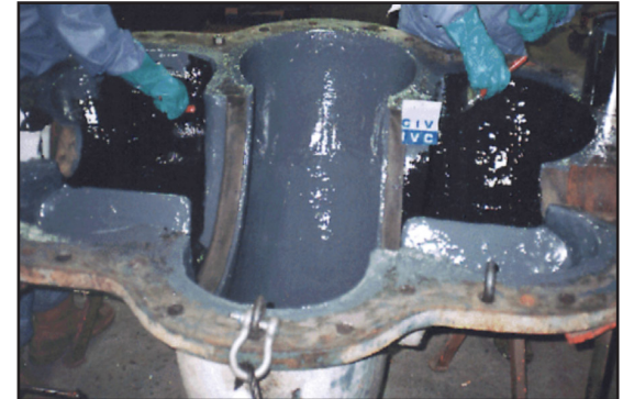
Final topcoat of ARC 855
