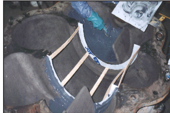
Re-building with ARC 858
